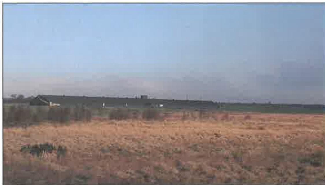
Fig 7: Poultry House 1km south of the appeal site on the same D17/1 road. (Typical in scale to the multiple others marked on aerial photograph)
